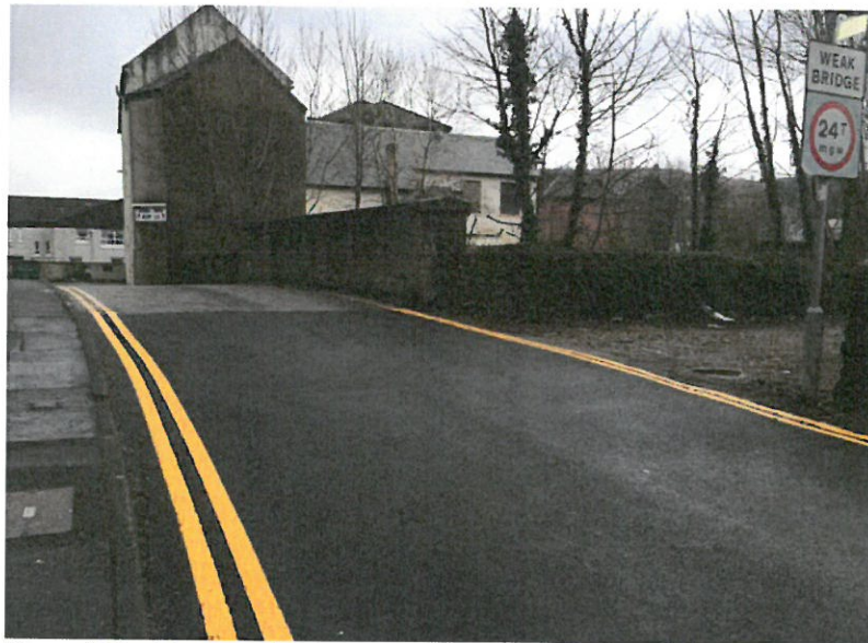
View of Site Entrance looking North East
